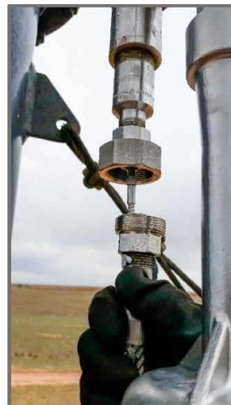
Figure 4 and Figure 5: Packaged fiber optic extension cable for vertical installation (left) and quick-connect expansion joint for modular installation in field assembly (right)
